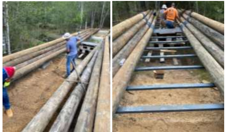
The 35' long poles were hoisted by chain with a mini trac hoe, steered along the path by the crew, and guided into the fabricated cradle.
