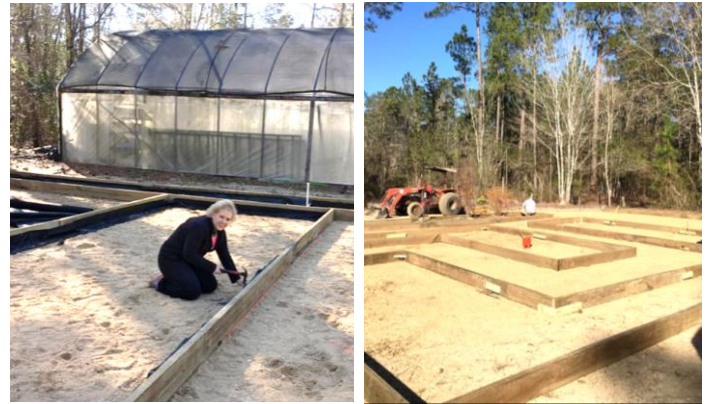
Michelle Berdux installs fabric in the new beds. The Partners crew has removed all of the existing materials in the Children's Garden, and we look forward to their planting project in April!
